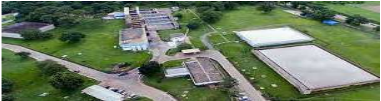
Figure 2: LWB Water Treatment plants
