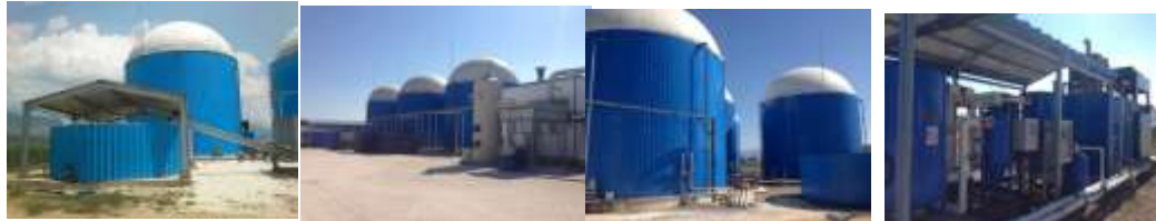
Figure 2 Homogenization tank, digester tank
